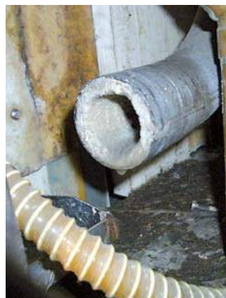
Pipe cross-section before
